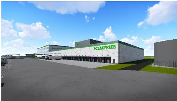
SCHAEFFLER is building a 61,000 m<sup>2</sup> logistical plant on a 145,000 m<sup>2</sup> plot of land, which will allow for the building's future expansion by up to 50%. The project comprises two 8,000 m<sup>2</sup> manual kitting areas on two floors of 8,000 m<sup>2</sup> each, served by a 7,500 m<sup>2</sup> DEMATIC Multishuttle area on the ground floor, a 39-meter high bay storage area, as well as 2,400 m<sup>2</sup> of offices.
